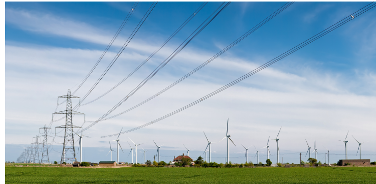
Cables conveying electricity
